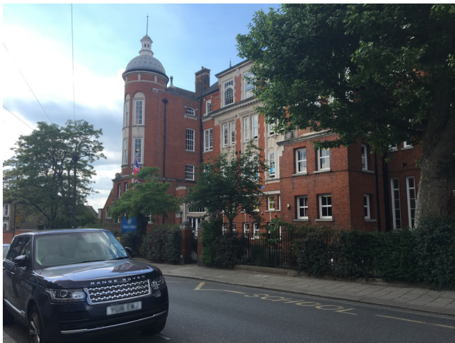
Figure 3. Building identified as the location of the interference source
