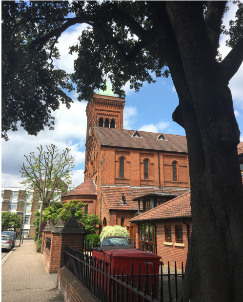
Figure 2. Church building housing the base station
